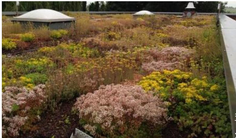
Extensive green roof
